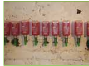
Automatic installation of the horizontal barrier
