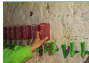
Installation of the cartridges
