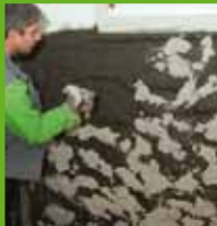
Application of the KÖSTER plaster key
