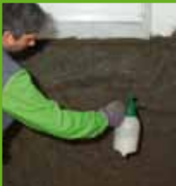
Priming with KÖSTER Polysil® TG 500
