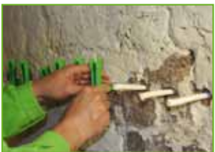
Installation of the KÖSTER Suction Angles
