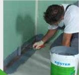
The fabric edges of the KÖSTER BD Flex Tape K 120 are overworked so that the fabric is completely covered with KÖSTER BD 50.
