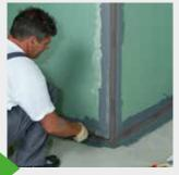
The KÖSTER BD Flex Tape K 120 forms a crack-bridging connection of the area waterproofing from wall to floor. It is installed in wall / floor junctions and over inside and outside corners.
