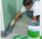
The area along the wall-floor transition is prepared with a layer of KÖSTER BD 50, which should cover approx. 10 cm of the wall and 10 cm of the floor.
