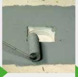
The surface onto which the KÖSTER BD Floor Sleeve is to be applied must be prepared with a layer of KÖSTER BD 50.
