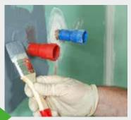
The fabric edges of the KÖSTER BD Wall Sleeve are overworked so that the fabric The KÖSTER BD Wall Sleeve is embedded is completely covered with KÖSTER BD 50.
