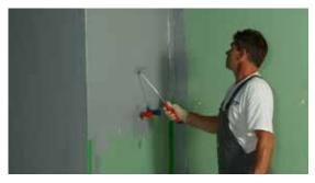
KÖSTER BD 50 is applied with a brush or roller. Waterproofing layers are always applied in at least two layers. The total consumption is approx. 1.2 kg/m<sup>2</sup>. The waiting time between the individual layers is at least 3 hours.
