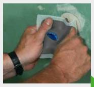
The KÖSTER BD Wall Sleeve is pulled over the end of the pipe.
