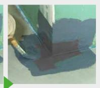
The fabric edges of the KÖSTER BD Outside Corner are overworked so that the fabric is completely covered with KÖSTER BD 50.
