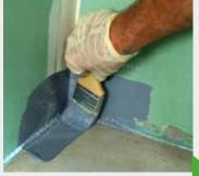
The corner is first prepared with a layer of KÖSTER BD 50, which should cover approx. 10 cm of the wall and 10 cm of the floor.
