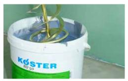
Prepare the KÖSTER BD 50 First, KÖSTER BD 50 is stirred in the bucket for approximately one minute using a slowly rotating electric mixer (below 400 rpm).
