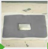
A hole in the shape and size of the floor drain is cut in the KÖSTER BD Floor Sleeve. Please note that the KÖSTER BD Floor Sleeve should overlap approx. 3 mm inwards into the floor drain.
