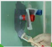
The area around the pipe penetration is prepared with a layer of KÖSTER BD 50. in the still fresh layer of KÖSTER BD 50.
