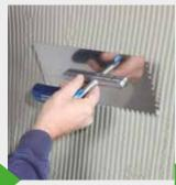
After the waterproofing is completely cured, the KÖSTER BD Flexible Tile Adhesive is applied with a notched trowel. The consumption depends on the tile size used. Detailed information can be found in the Technical Data Sheet.
