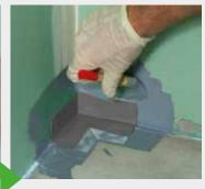
The fabric edges of the KÖSTER BD Inside Corner are overworked so that the fabric is completely covered with KÖSTER
