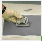
The KÖSTER BD Floor Sleeve is positioned above the floor drain.
