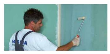
Application of the KÖSTER BD 50 Primer KÖSTER BD 50 Primer is applied to the substrate with a brush or roller. The consumption varies depending on the type of substrate, between 50 – 150 g/m<sup>2</sup>. For more detailed information on other substrates, please refer to the Technical Data Sheet.
