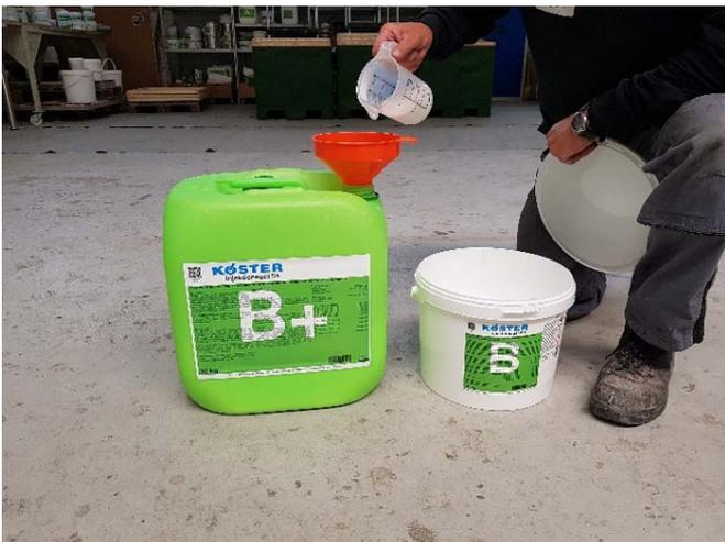
The mixed components can be processed for 2 hours.
